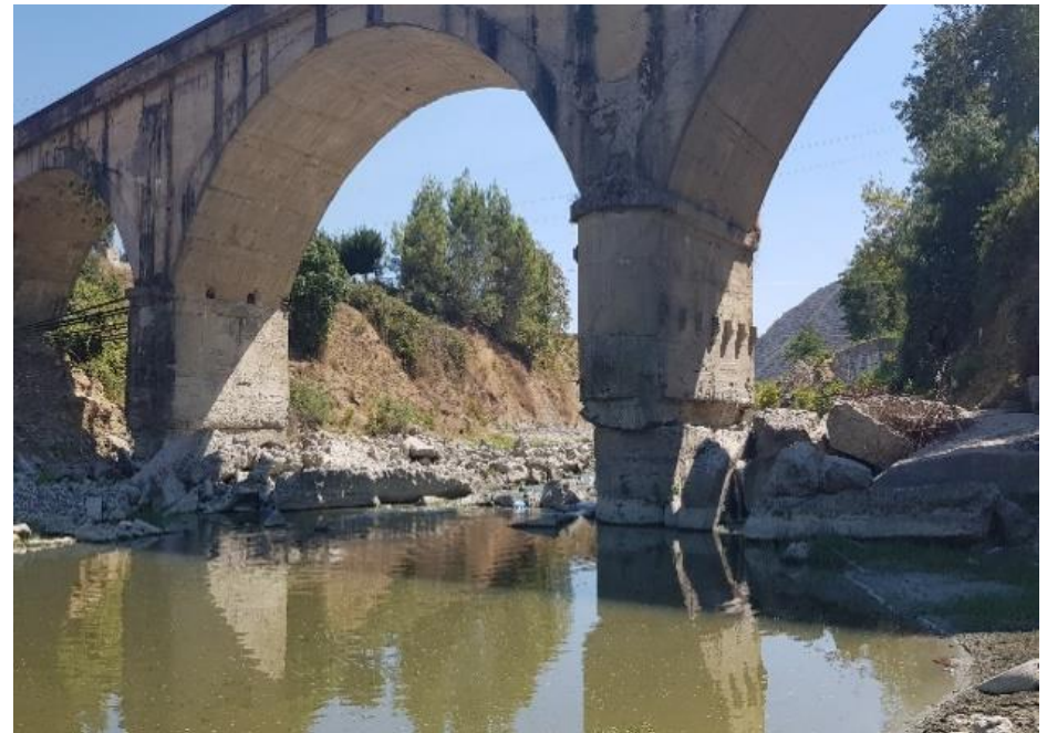
Evidence of incision in a bridge of Erzen River, 2020
